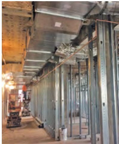
PHOTO: Renovation work at Baldwin Hall at Truman State University
